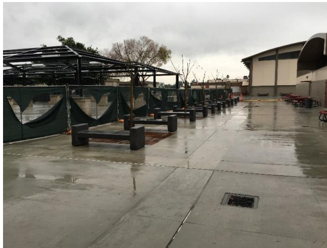
New Seating Near Area D1
