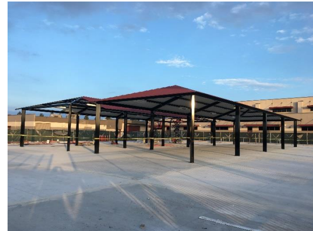
Shade Structures at Area C2
