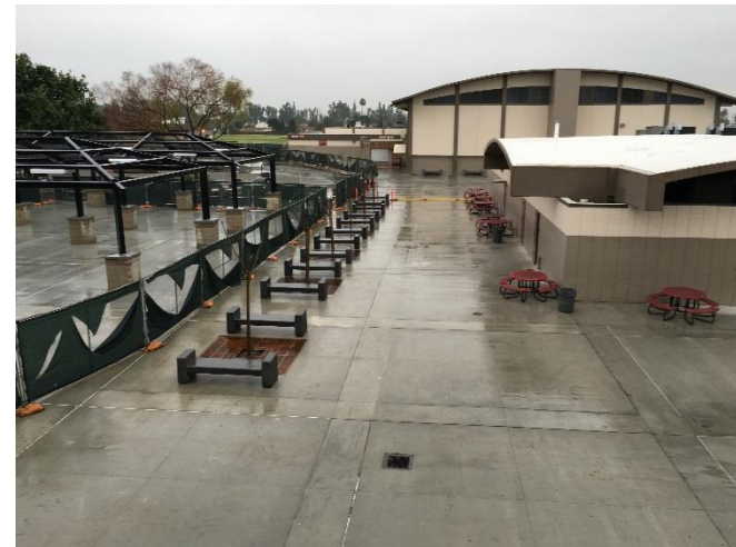
New Seating and Shade Structures In Progress
