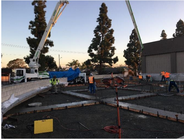
Concrete Infill Pour at Theater Courtyard
