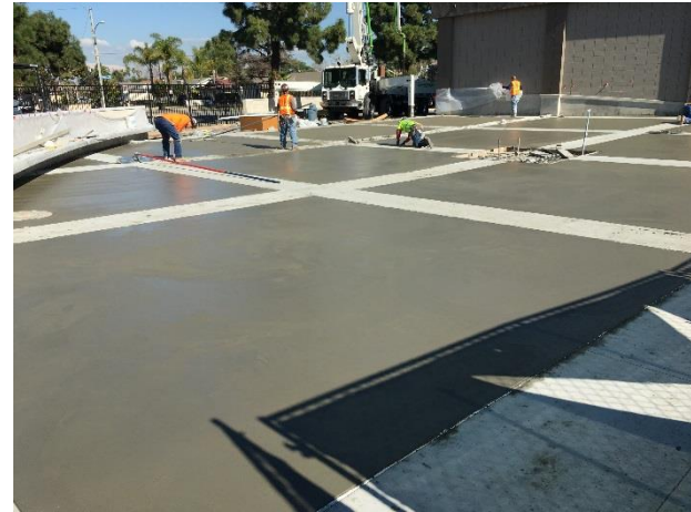
Concrete Infill Complete at Theater Courtyard
